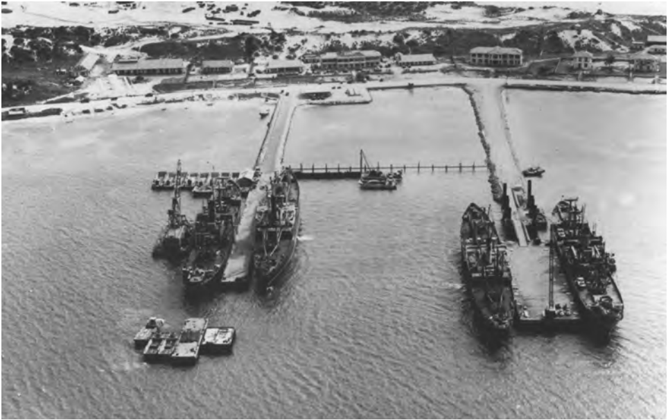
Deep-draft piers at Cam Ranh Bay in January 1966 showing the RMK pier built in 1964 at left and the recently completed DeLong pier and causeway on the right
